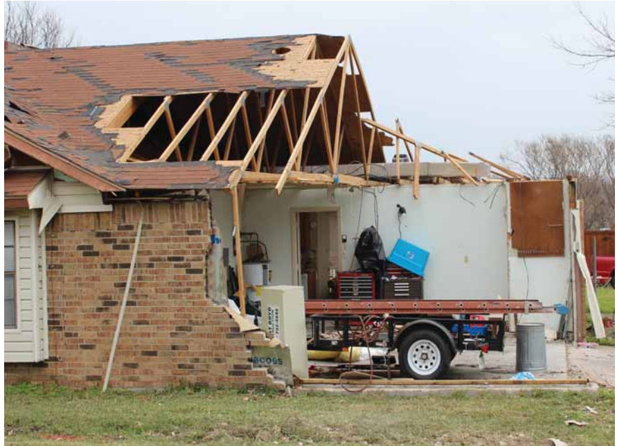
In this home in Rowlett, Texas, failures were initiated adjacent to large openings such as this garage door. Wind in this area was consistent with a rating of EF0 to EF1 based on the degree of damage to roof coverings and nearby trees. Garages are more vulnerable to damage since they are less structurally redundant and often lack adequate lateral bracing at the walls containing the large vehicular opening.
