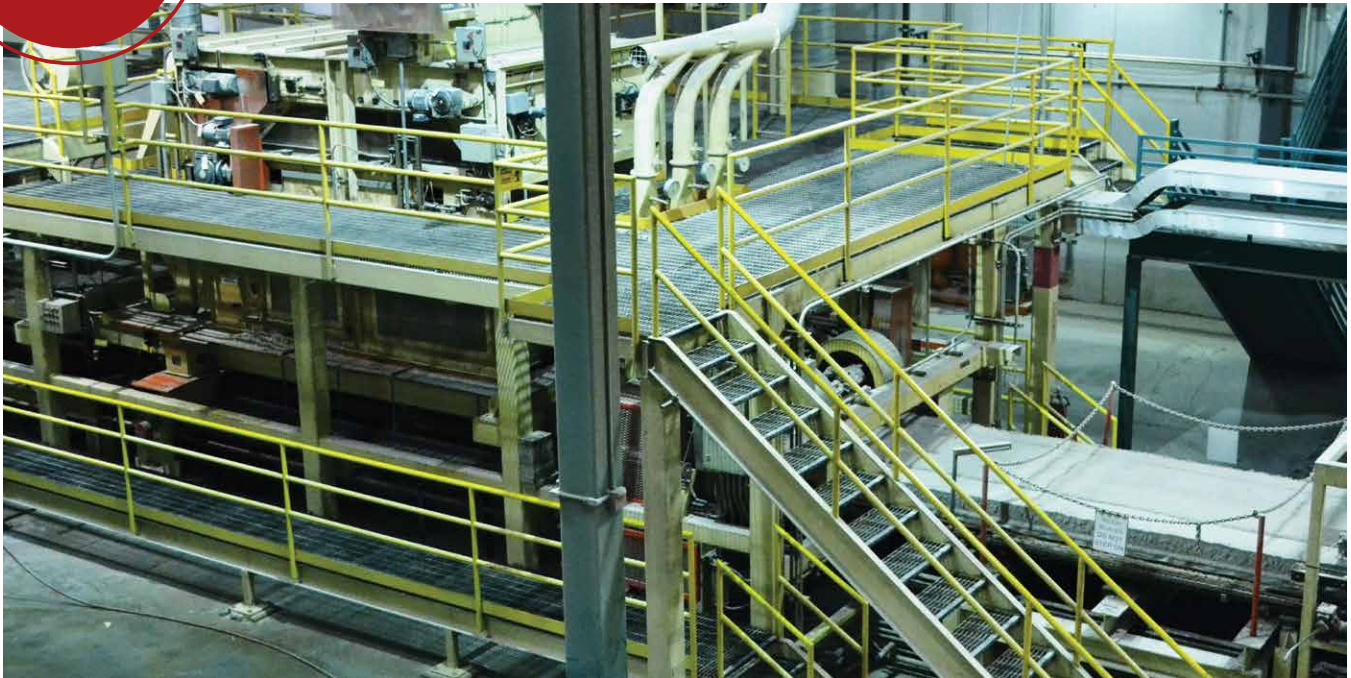
Image courtesy of Fiber Commercial Technologies
