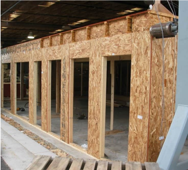
2006: APA Research Center full-scale single-story house test in process.
