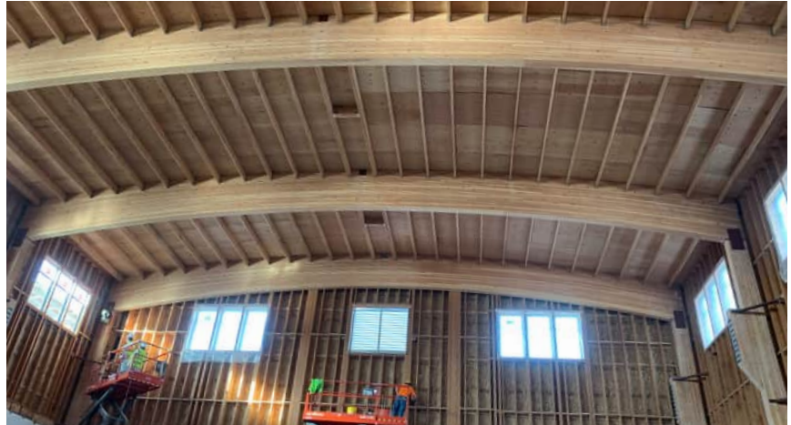
2019: Framing of the new APA Research Center high-bay laboratory
