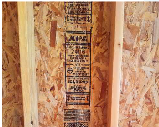
APA and APA EWS trademarks are the manufacturer’s assurance that the product conforms to manufacturing and product performance standards shown on the trademark.
