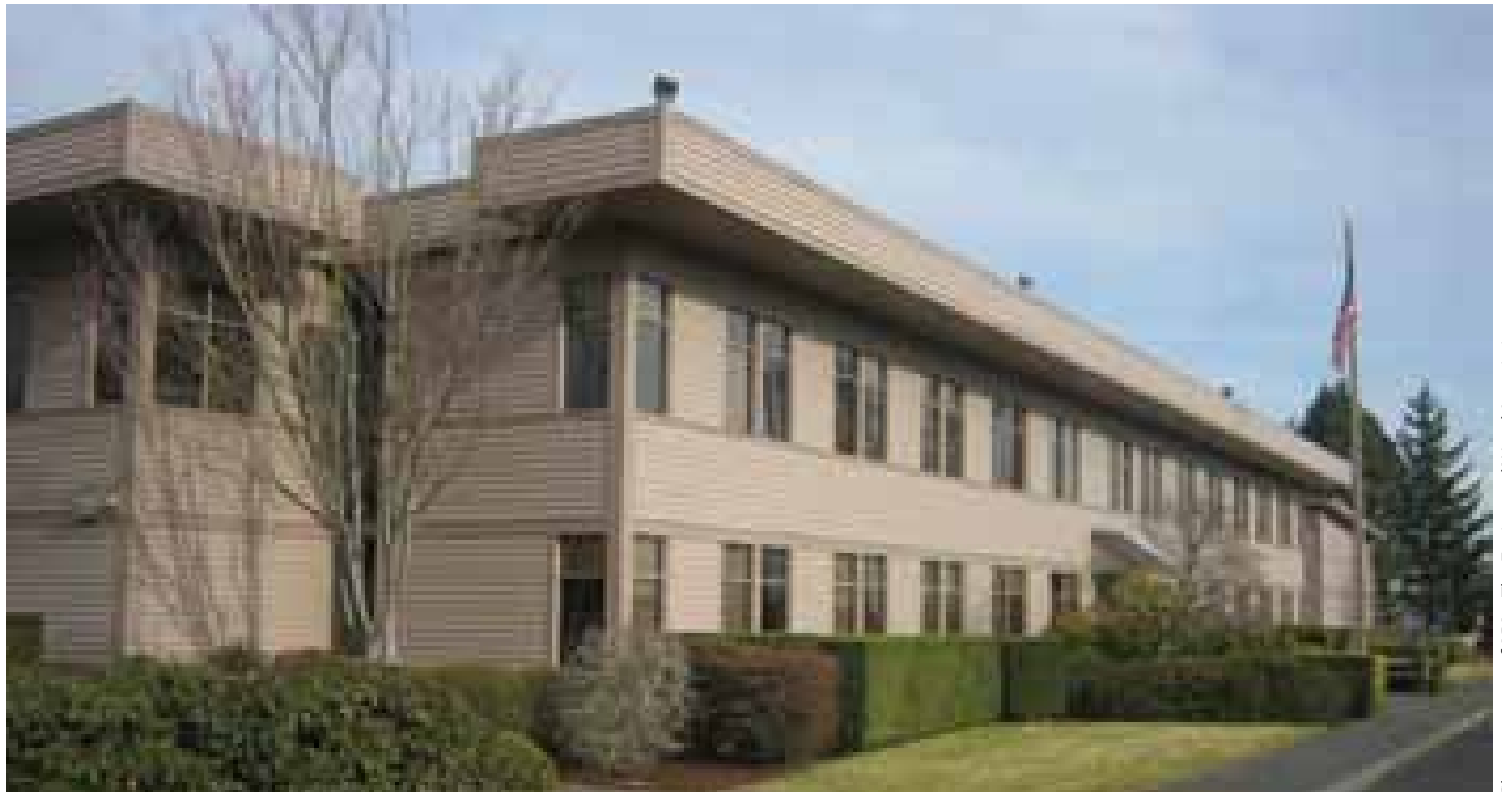
Opened in 1969, APA's 42,000-sq-ft Research Center in Tacoma, Wash., houses APA's Technical Services Division staff and a wide array of product and systems testing equipment.
